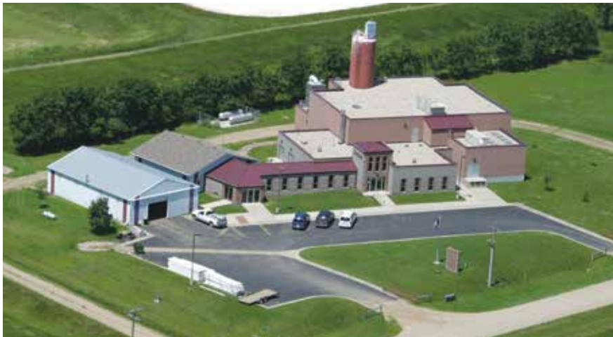
Big Sioux Community Water Headquarters in Egan, SD
