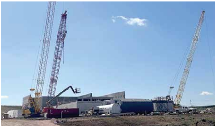
Progress photo of the Shared Resources plant near Trent, SD
